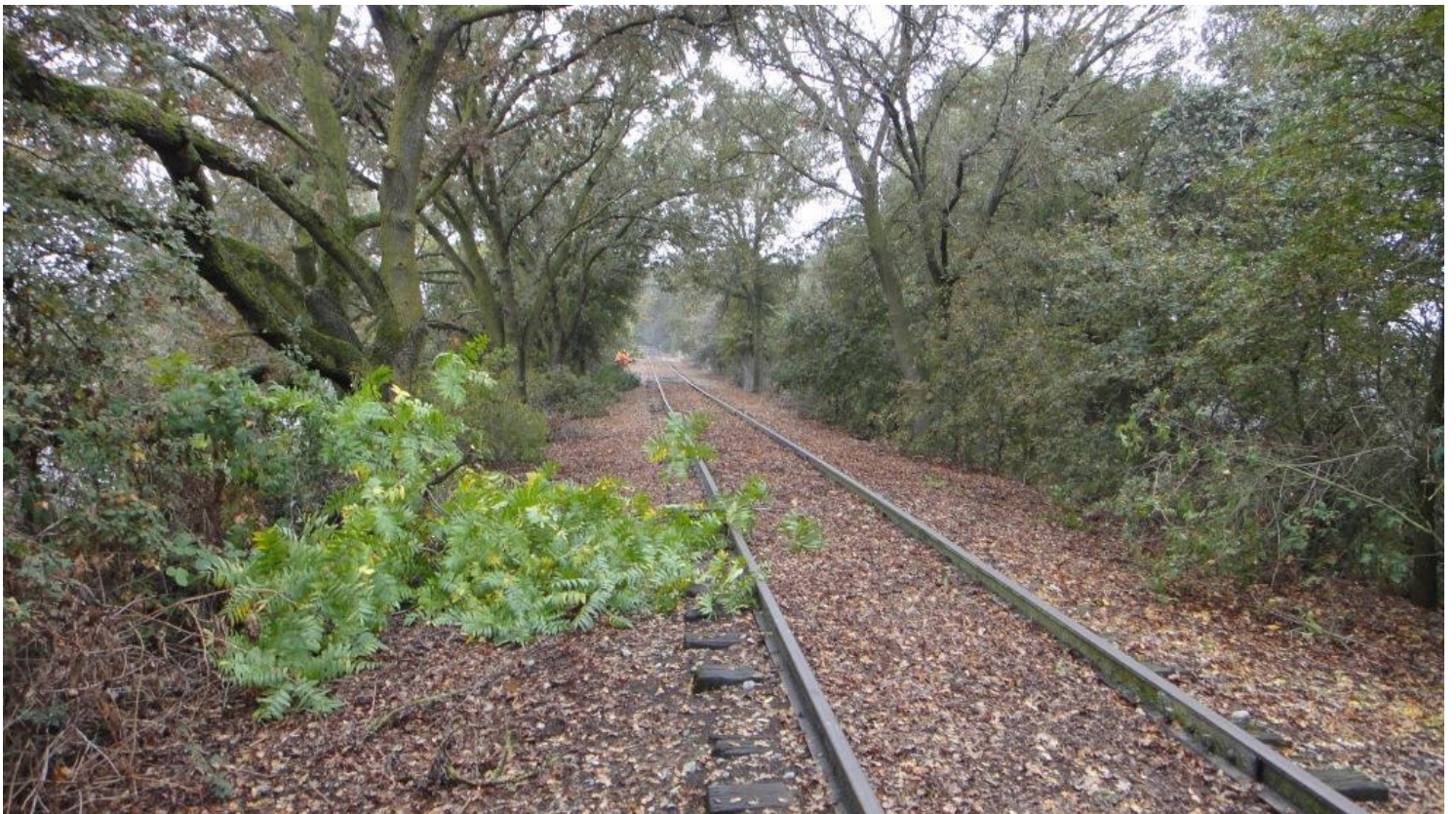
The picturesque Hood Line at Mile Post 12.1
