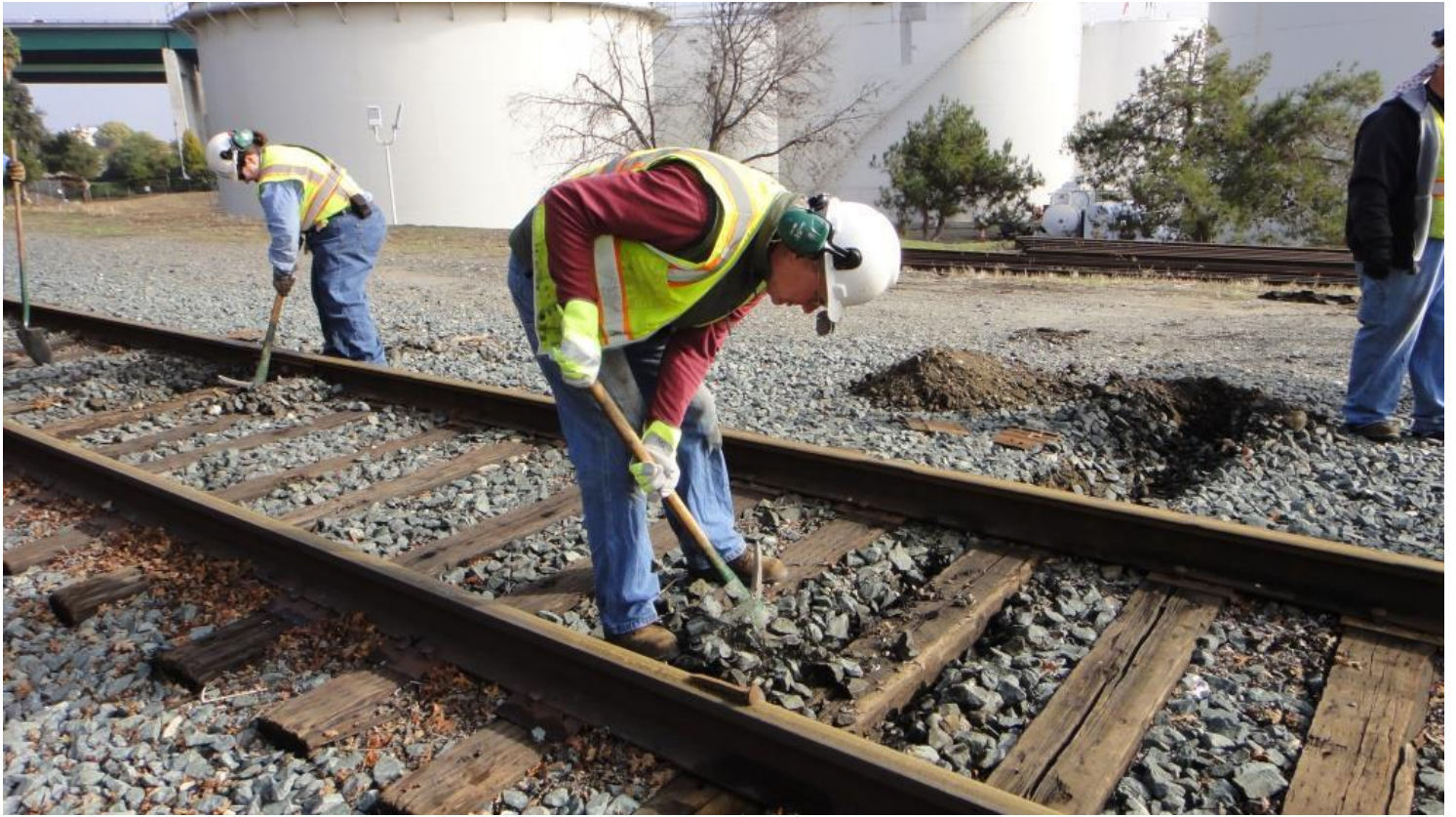
Heather and Steve digging out the sides of the ties
