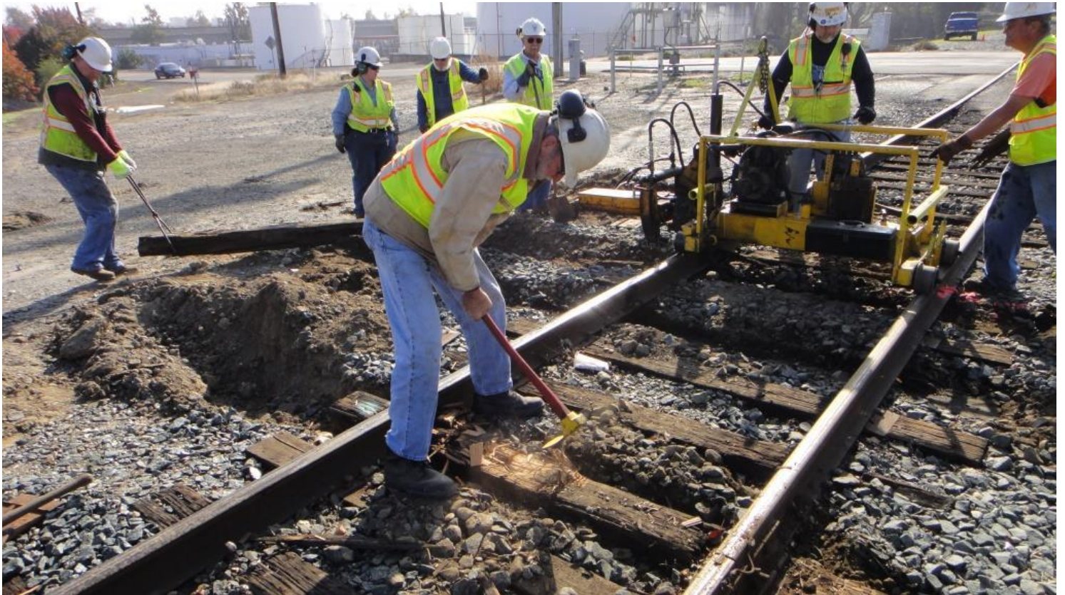
Alan adzes the top of a plate-cut tie
