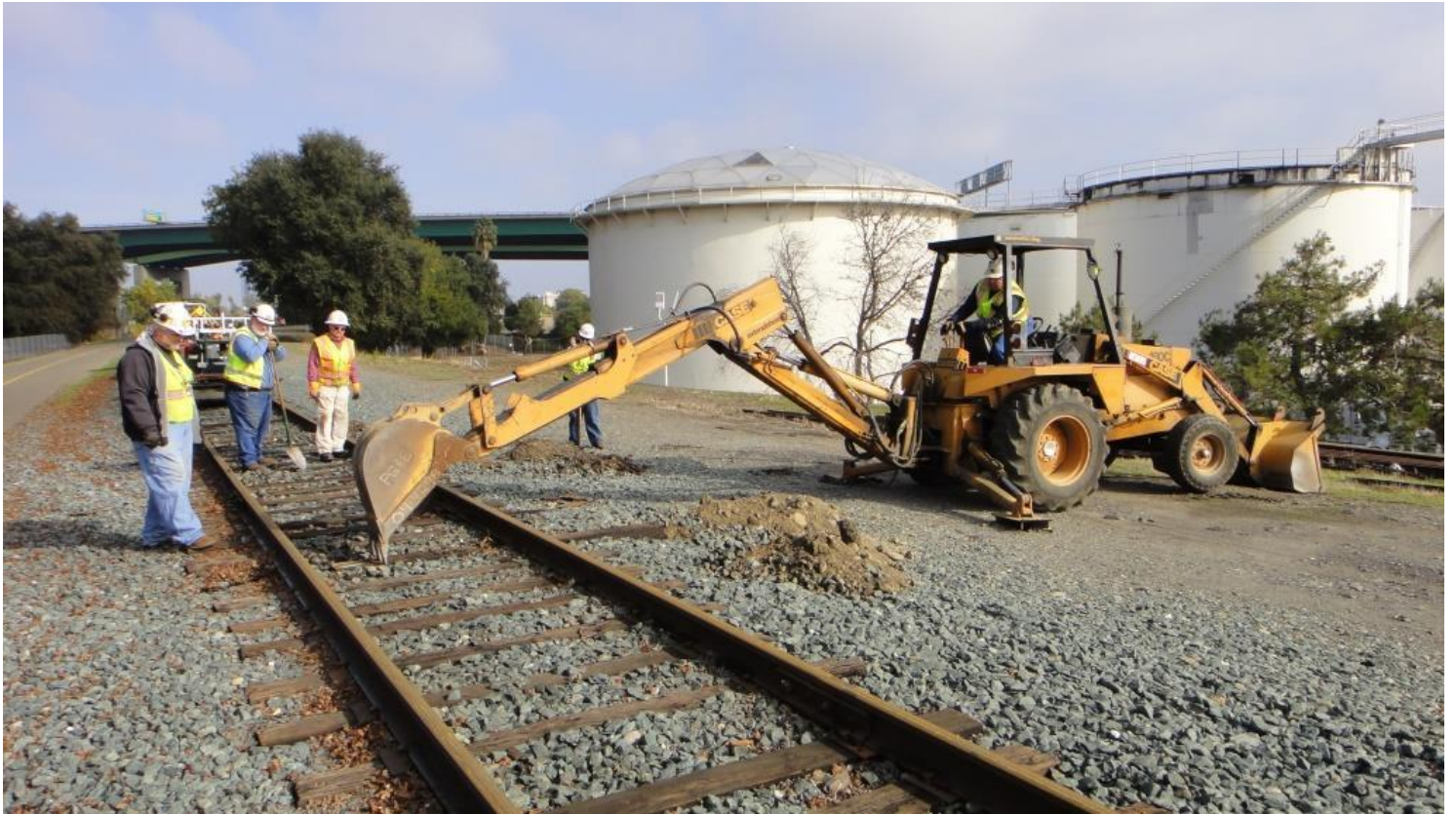
Harry brings in the back-hoe to pull a particularly stubborn tie
