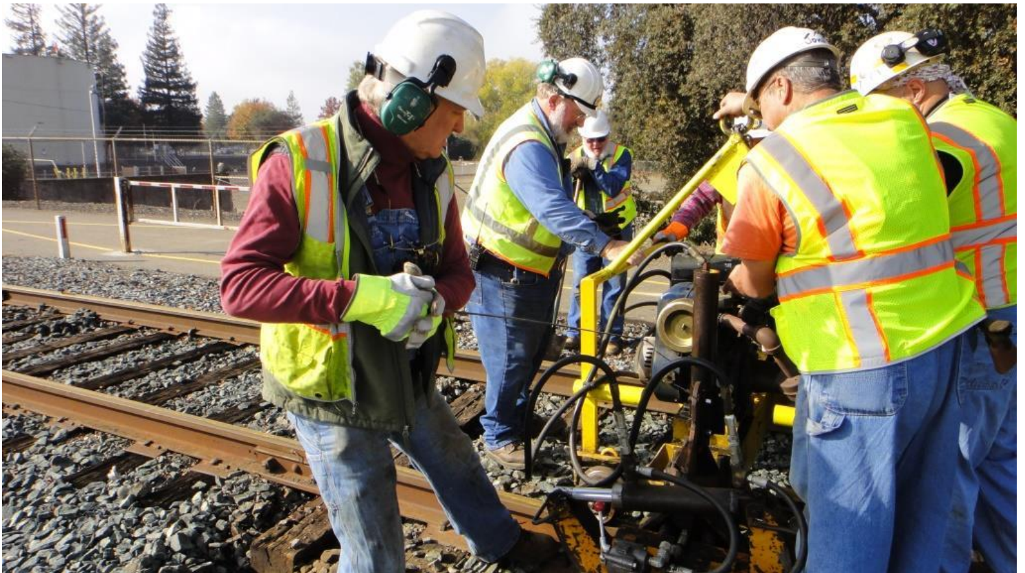
Steve powers up the section-gang machine
