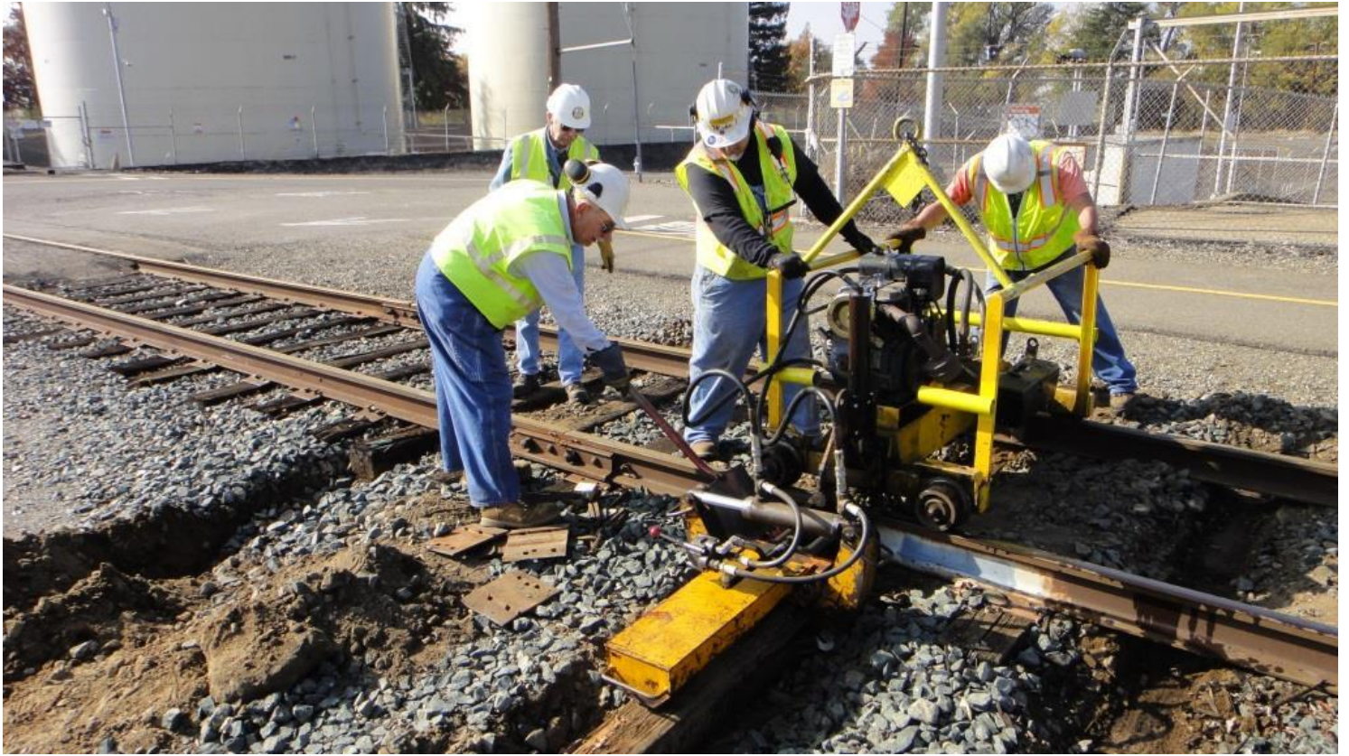
Signal Jim watches carefully as Mike F. and Clem pull a tie that runs right along the shunt
